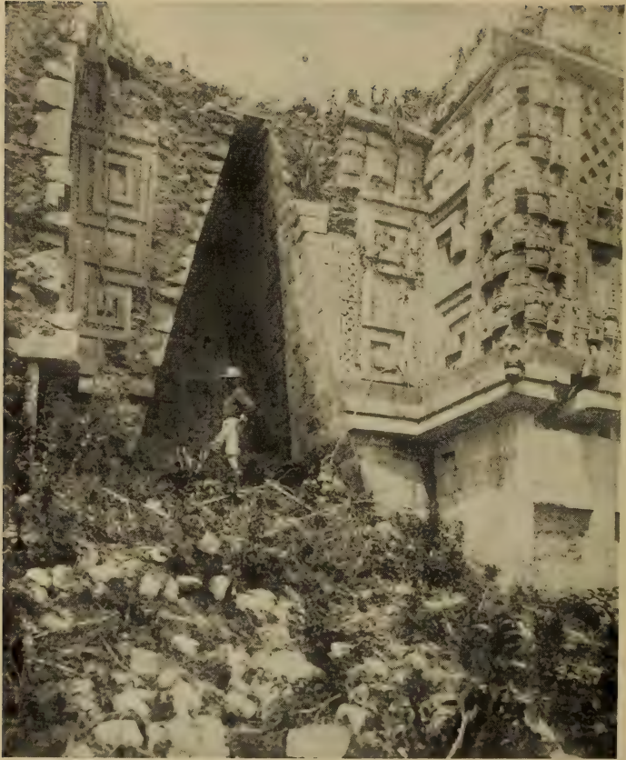
Plate XVII. A Sealed Portal Vault in the House of the Governor at Uxmal, a Building of the Second Empire, probably Thirteenth Century. The veneer character of the cut stone comes out clearly. Peabody Museum photograph.
